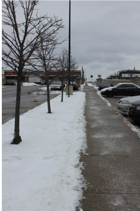
Figure 7-10 Salt applied to a sidewalk in the Lake Simcoe watershed. Salt applied in anticipation of freezing rain and freeze-thaw events can be harmful to nearby trees and shrubs.
