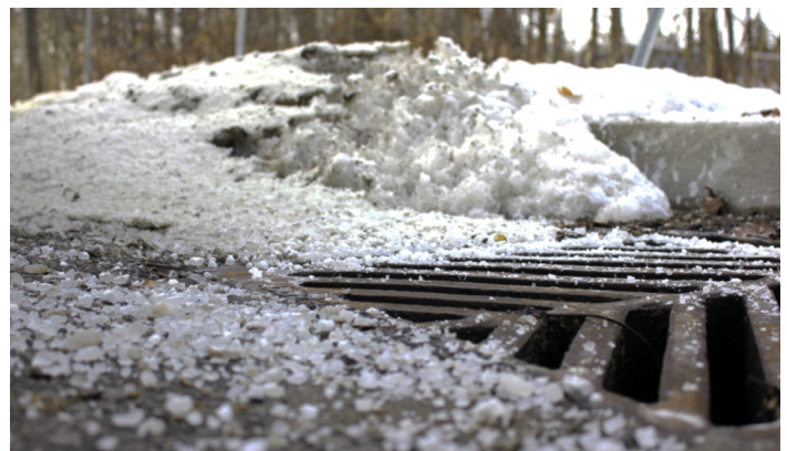
Figure 2. Salt over applied in a parking lot
