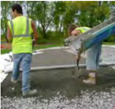
Left: Installation of pervious concrete; community recreation application. Right: Installation of permeable pavers.
