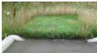
Turf blocking inlet (CVC).
