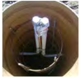
Lighting base installation.
