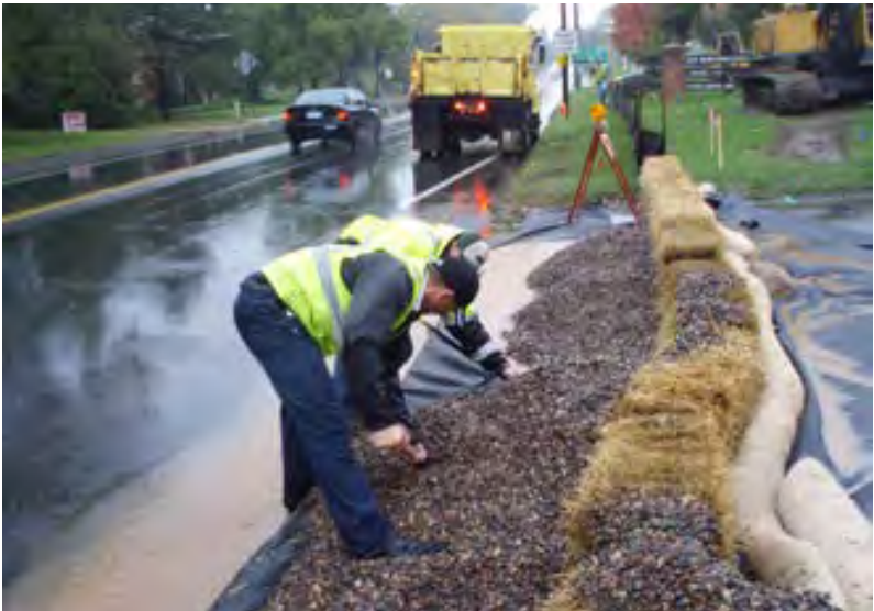
Emergency Erosion and Sediment Control.
