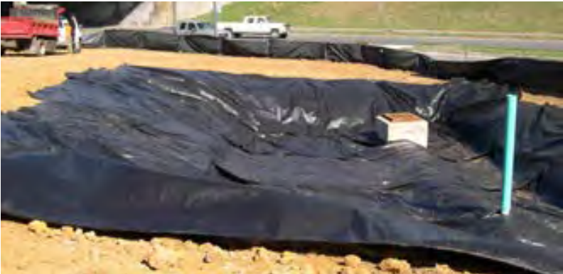
Image-silt fence incorrectly lining BMP (Source: LID Center).
