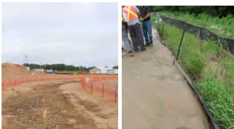
Left: Caution fencing prevents traffic and building materials storage within the BMP. Right: A double row of silt fence, the first row is on the verge of being overwhelmed and requires immediate maintenance.
