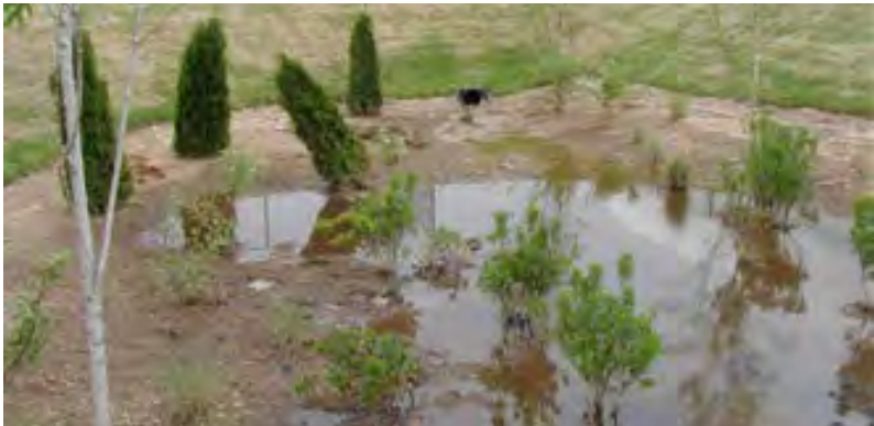
Bioretention clogged with construction sediment which could have been prevented with effective ESC implementation. Source: LID Center
