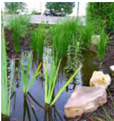
Left: BMP holding water longer than design drawdown time. Right: Double-ring infiltrometer.
