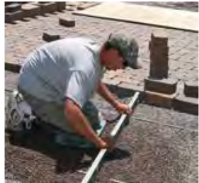
Left: Installation of pervious concrete; community recreation application. Right: Installation of permeable pavers.
