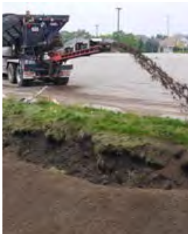
Slinger truck evenly placing bioretention soil in a large cell.
