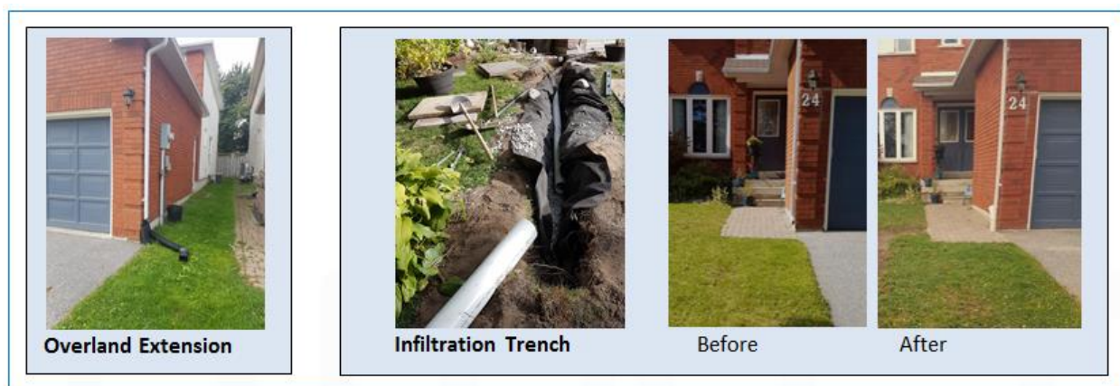
Figure 1: Two Types of Downspout Redirection Projects
