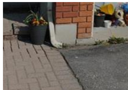
Figure 10: Pavement Slumping from Water Ponding at Base of Downspout
