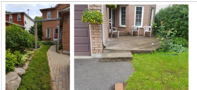
Figure 11: Creative Solutions for Dealing with Walkway Downspouts
