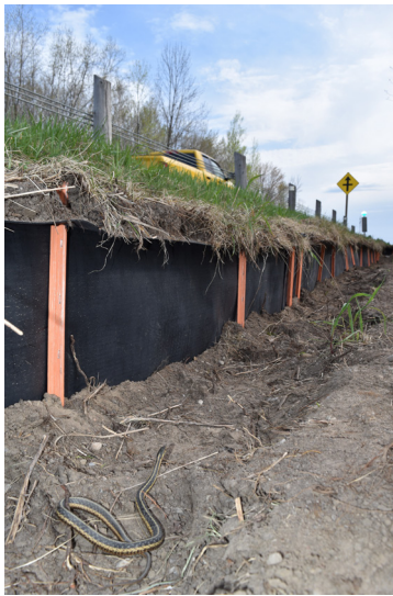
Garter snake safely excluded from the roadway by ecopassage fencing
