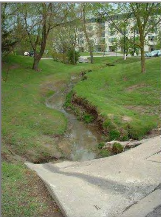
Figure 3-7: A project undertaken in an urban area in Newmarket to mitigate bank erosion and create a naturalized stream channel and fish habitat. Photos show the channel before the project was initiated (top left), during construction (top right), and after construction (bottom right)
