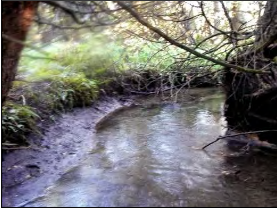
Figure 7-7: Pefferlaw Brook Reach PB50-6: scouring of banks.
