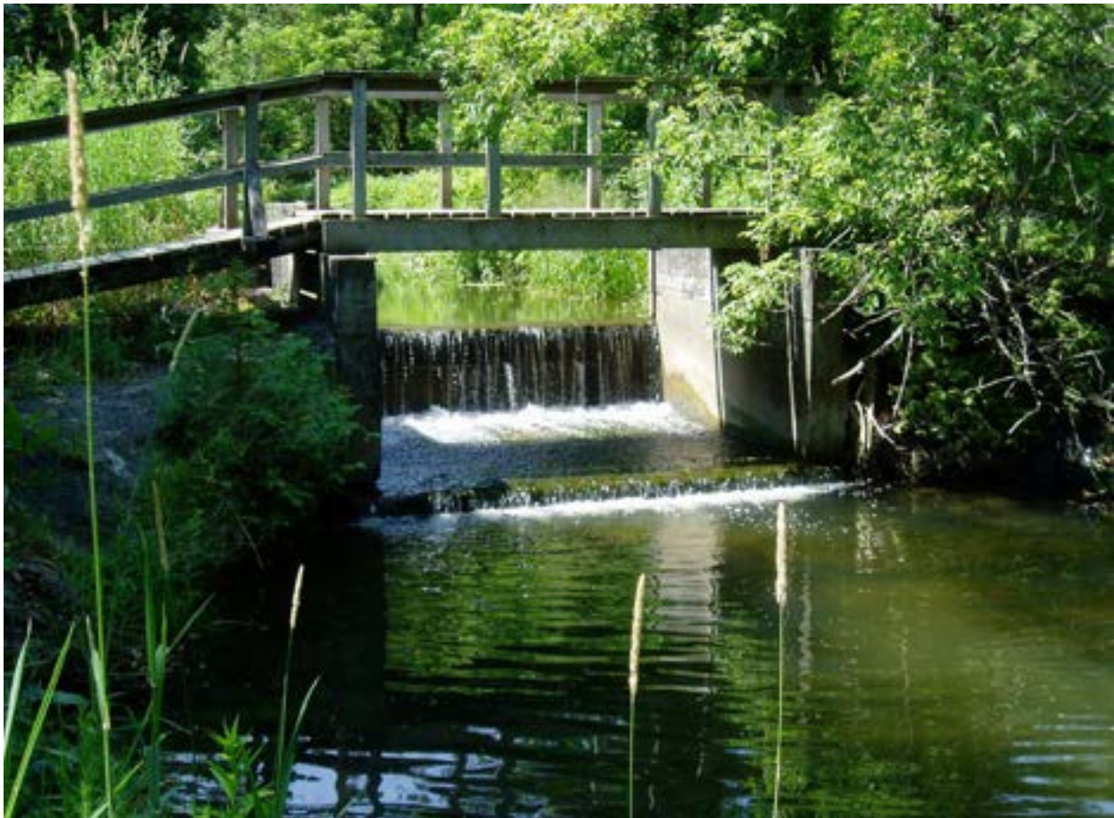
Figure 6-4 The Camp Kettleby Dam – An example of an on-line structure within the West Holland River subwatershed
