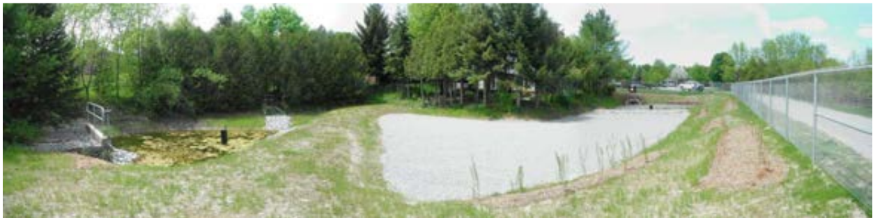
Figure 11 - Overview of facility post-construction
