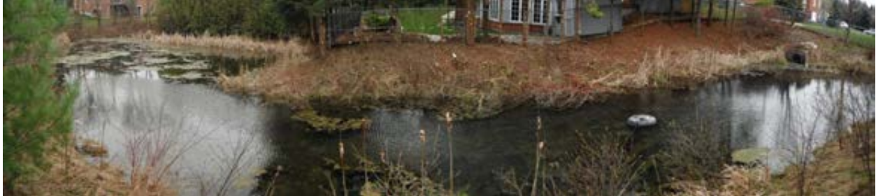
Figure 10 - Overview of facility pre-construction
