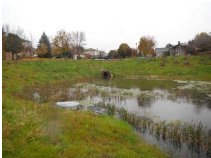
Figure 9 - Colony Trail wetland, outlet structured in foreground, inlet structure in background
