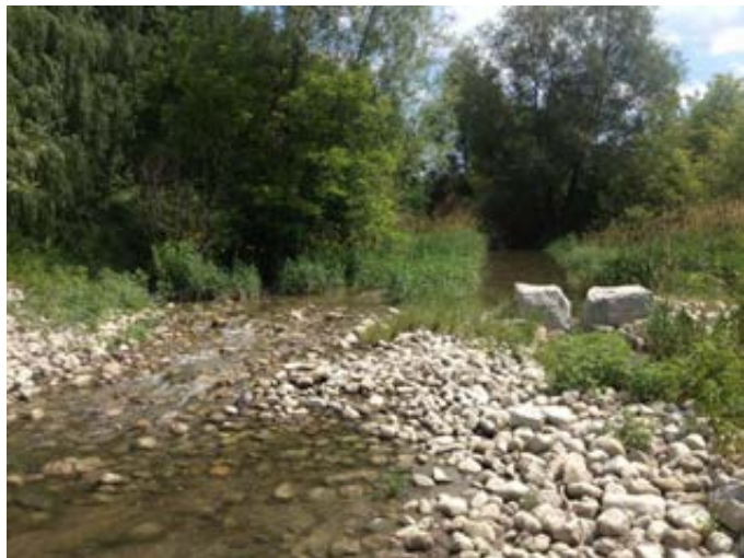
Figure 2 - Inlet Channel to George Richardson Pond showing stone flow splitter and By-pass Channel on right
