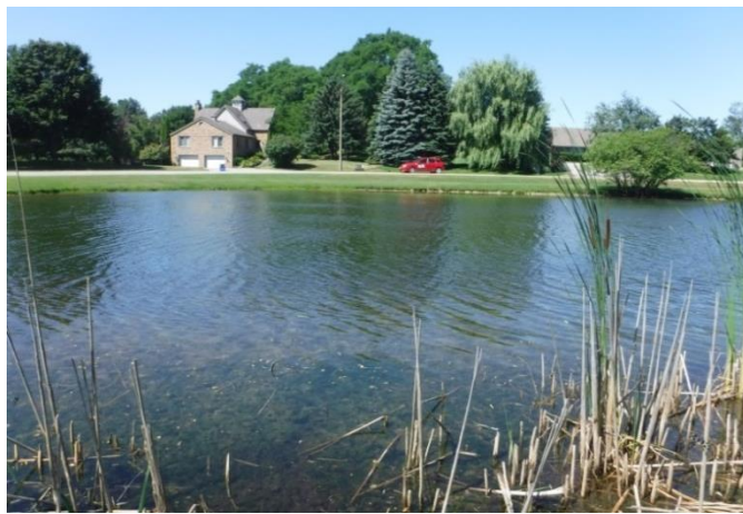
Figure 5: Stormwater pond in good condition
