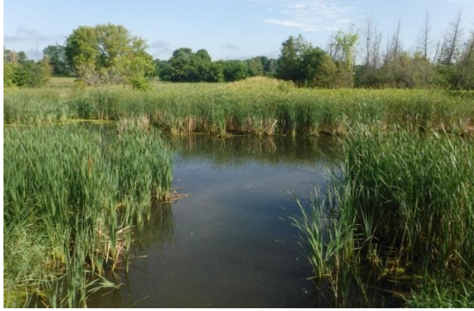
Figure 4: Stormwater pond in good condition
