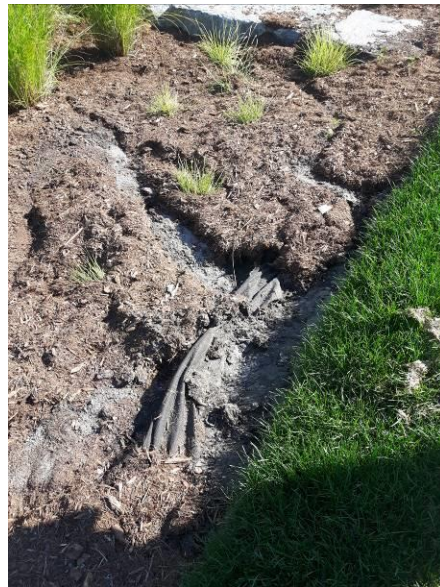
Figure 14: A bioswale with exposed bio filter and significant erosion of the top soil layer
