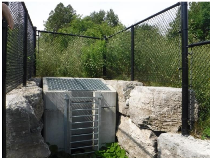
Figure 6: Stormwater pond outlet in good condition
