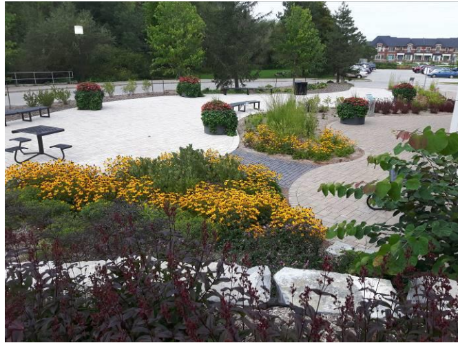
Figure 11: Rain garden and permeable pavement
