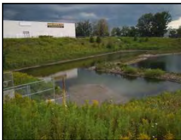
Stormwater Pond – BAR-SW42
