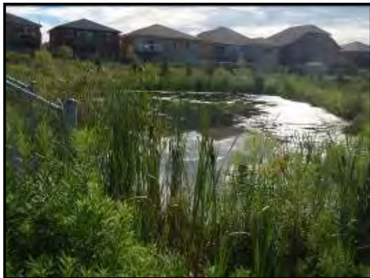
Stormwater Pond – BAR-SE86
