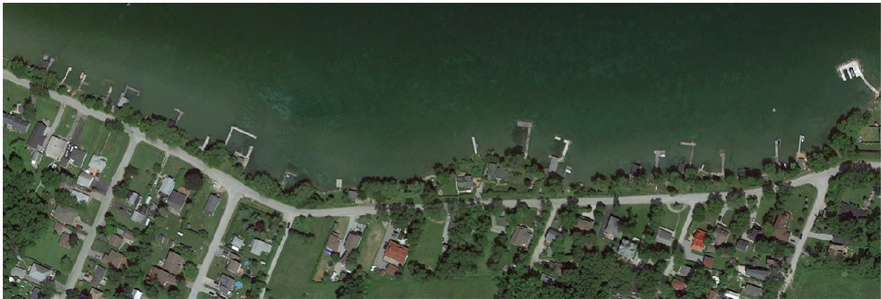
Figure 9.4: Offshore Breakwaters Along Shore South of Snake Island
