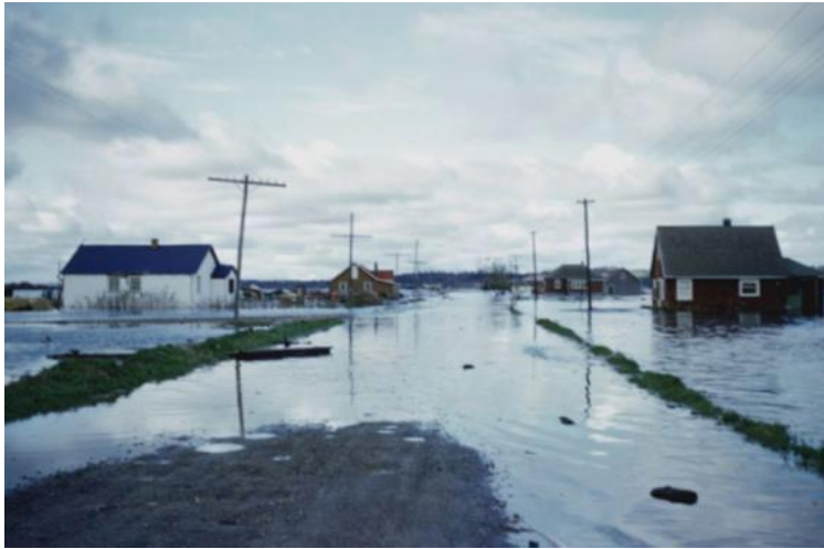
Figure 10: Flooding within the Holland Marsh as a Result of Hurricane Hazel (October 1954)
