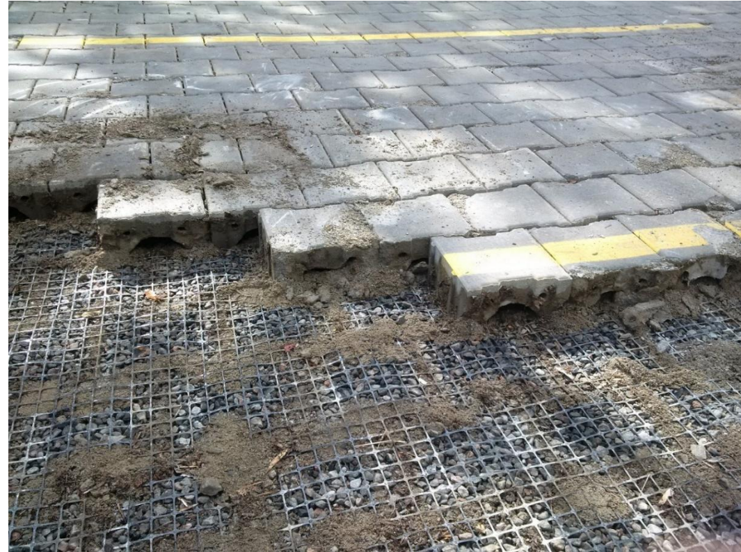
Permeable Blocks Crumbling in 2018 (2 years Post-Installation)
